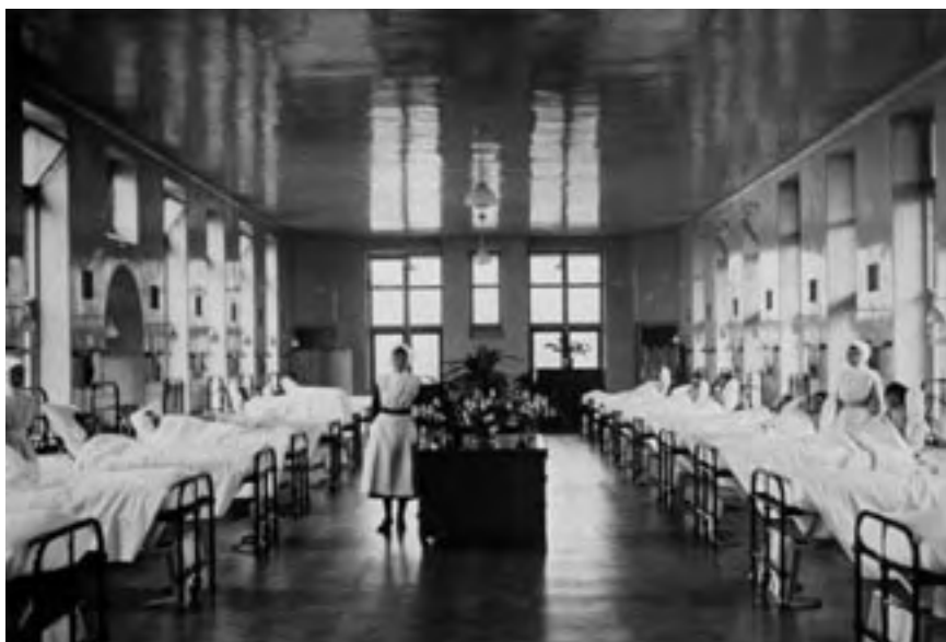
Figure 7. Interior, Nightingale Ward, circa 1930, Darlington Memorial Hospital. [Copyright: Wellcome Institute Library]
