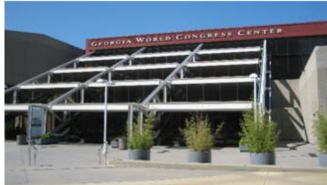
The entrance to the Georgia World Congress Center in Atlanta Courtesy of Ashley Judy
