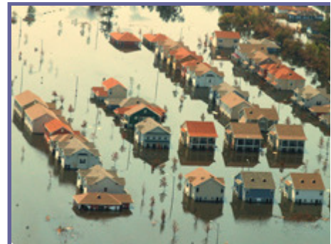
Photo courtesy of FEMA. This picture shows actual disaster site w conditions and may not illustrate proper and health procedures.
