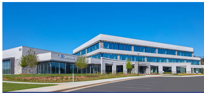
GreyStone Power's new corporate headquarters located on Hwy 92 in Paulding County opened March 2021.
